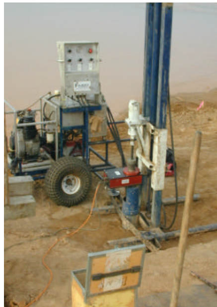
Figure 6: Pushing frame used for shear vane testing – also for piezocone probing
