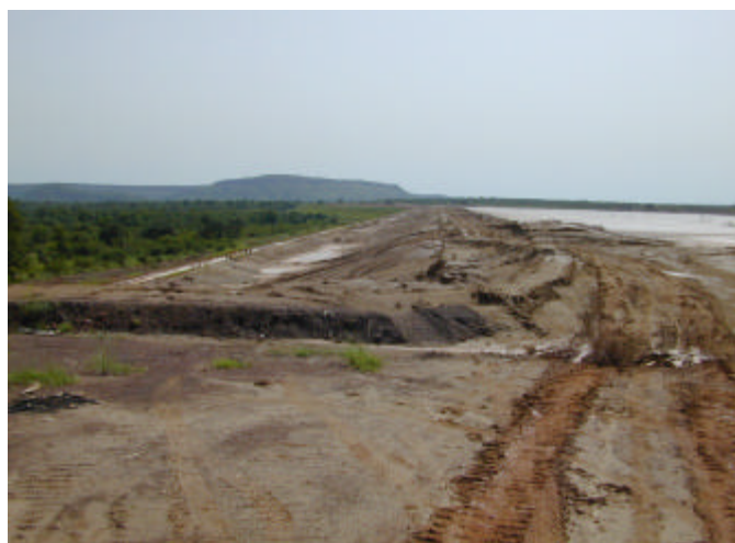
Figure 4: Sadiola deposit showing cycloned upstream raising (Sept. 2001)
